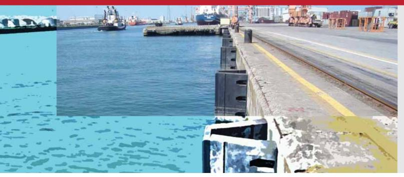
Arch and element fenders have been successfully used across the world for many decades already. The relatively simple and very strong construction and durable rubber quality of these fenders provide very good protection for quay walls and corners.
